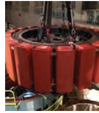
KAPLAN BLADE LOWERING AND INSTALLATION
