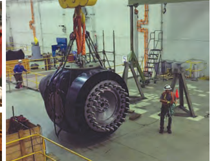
RUNNER HUB LIFTING AND INSTALLATION
