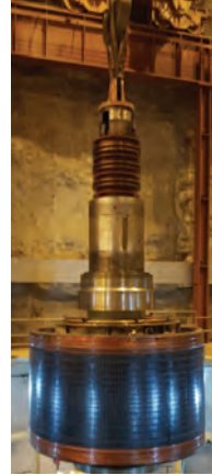
RUNNER HUB LIFTING AND INSTALLATION
