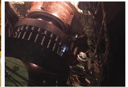
RUNNER HUB LIFTING AND INSTALLATION
