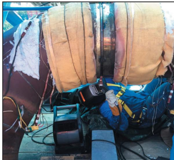
First time quality welding of the P21 and P22 pipe welds under controlled preheat.
