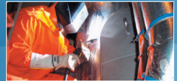
Specialty Welding & Machining
